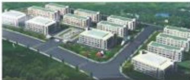
Hunan Jiaozuo West Industrial Area
